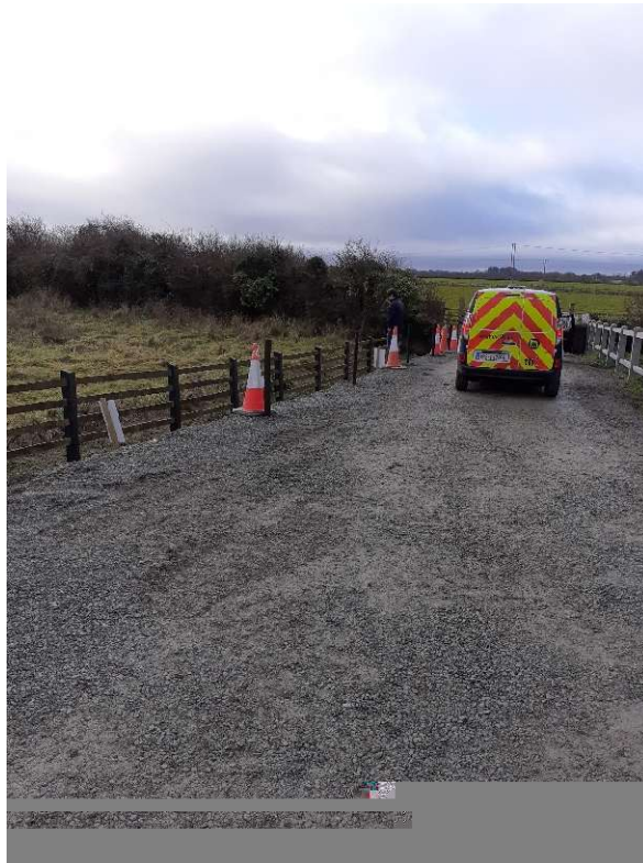
Figure 3: Crushed Rock Roadway
