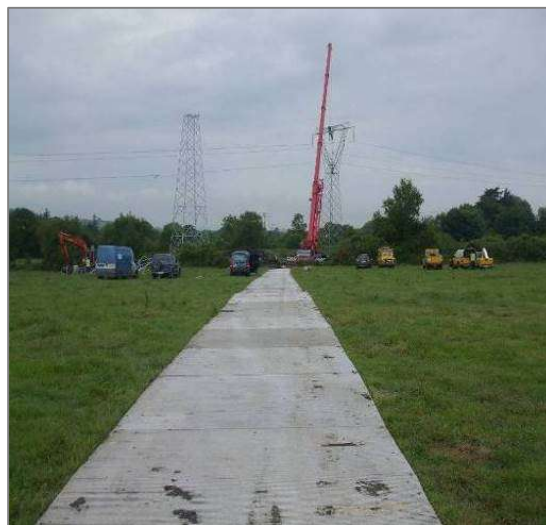
Figure 2: Temporary Aluminium Panel Tracks
