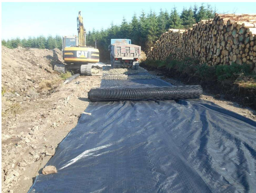
Figure 4: Crushed Rock Roadway Build-up With Geotextile
